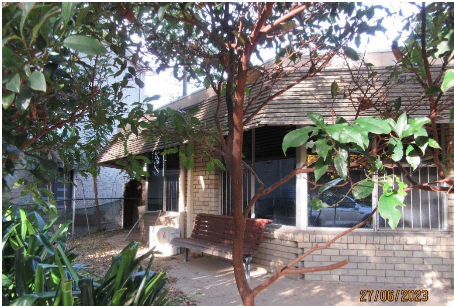
17 General view of the western side of the building.
