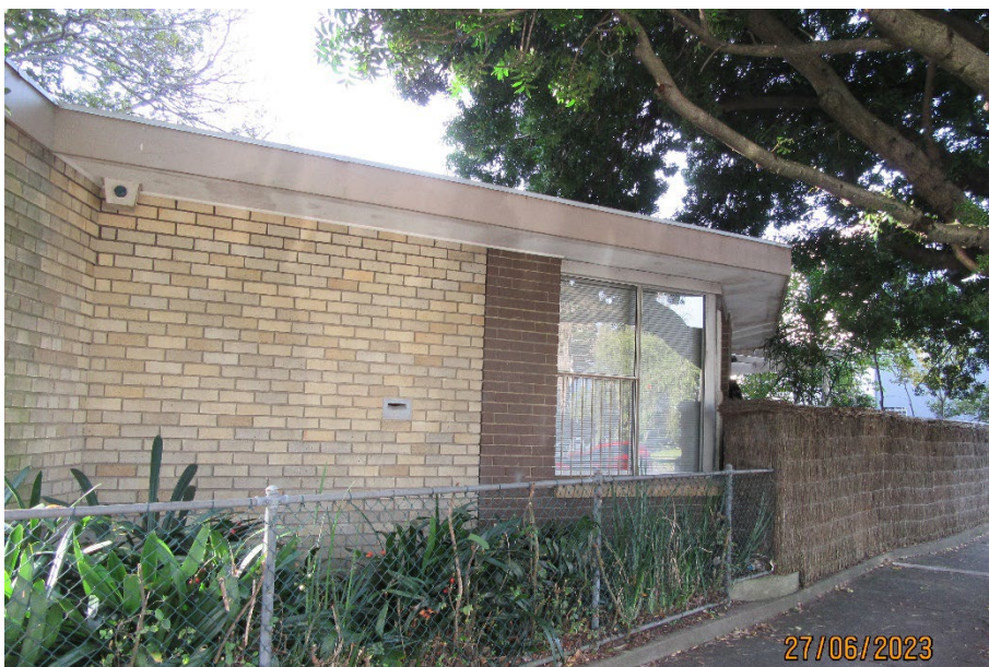
18 Looking along the side of the building facing Allen Street. Brush fencing encloses the yard at the rear of the site.
